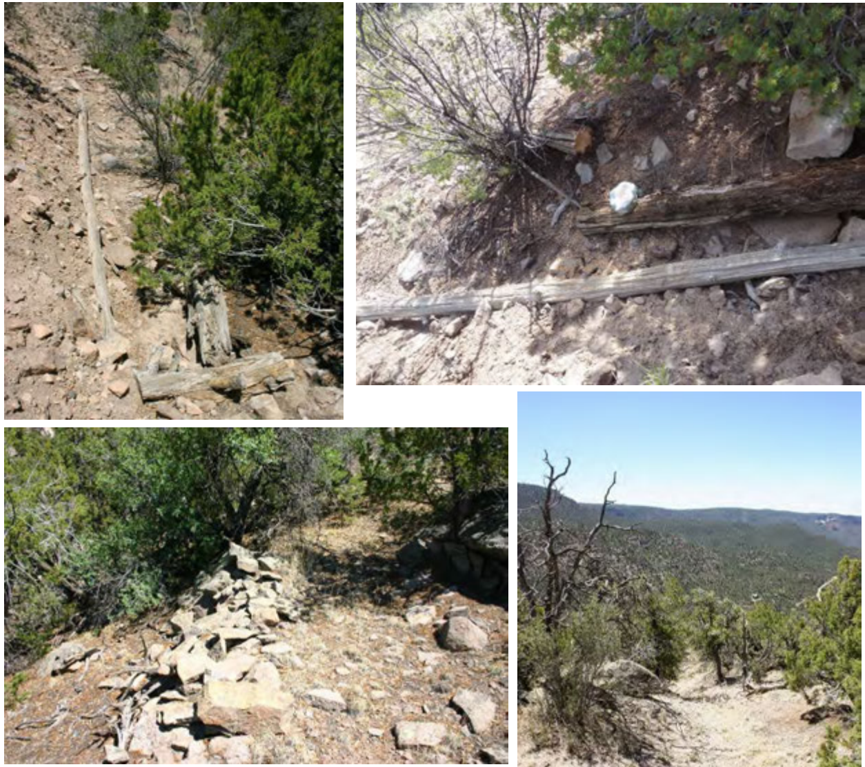
FIGURE 7. Upper left: A chute stick and two cross ties. Upper right: Sample LGC4 of a chute stick. Lower left: The rock cribbing below the chute path about half-way down the chute. Lower right: an entrenched portion of the chute path.
