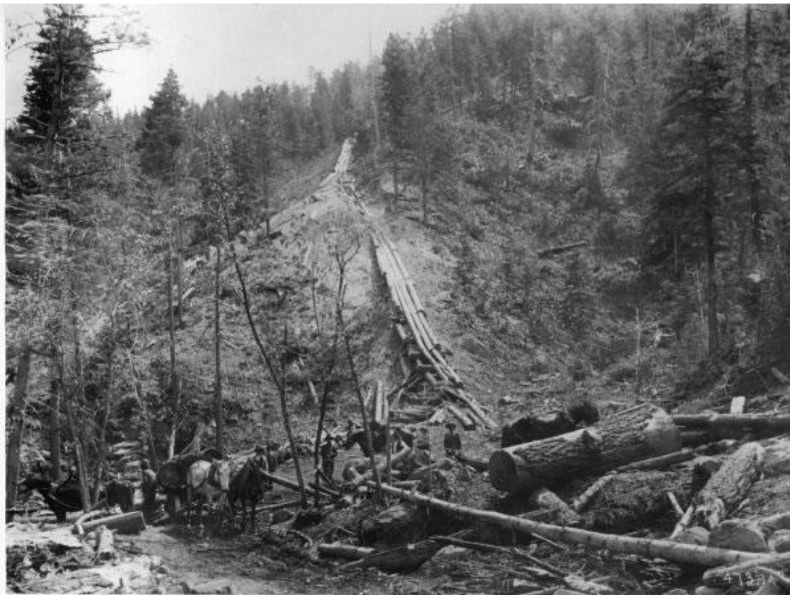
FIGURE 4. Log chute in Mediodia Canyon, Dye Timber Company circa 1910.
