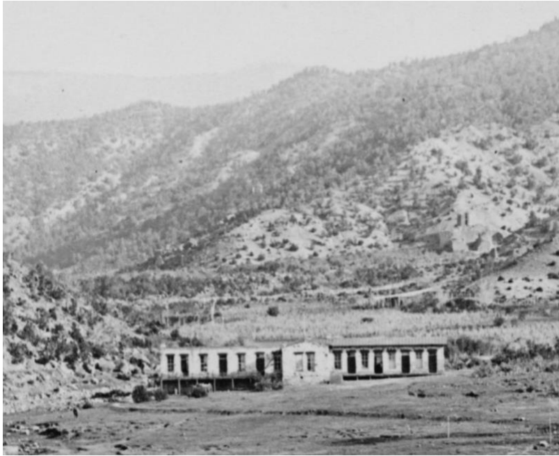
Figure 4. Zoomed in view of the old hotel and current building. Notice that part of the westernmost wing of the hotel is missing in the current building. Did a flood take out that part of the building? Also, notice the old mission church is visible right center in the distance.
