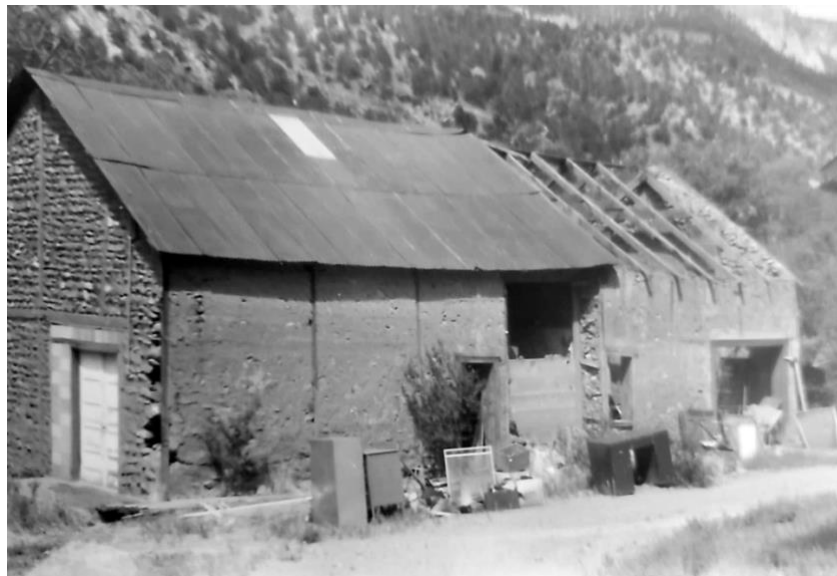
Fig. 9. Photograph of the barn immediately behind the Adams House, probably mid-twentieth century, supplied by Paul Adams, Jr. The barn was demolished soon after they traded the property; the Douglas-fir timber recovered from its footprint (Barn 1) was cross-sectioned and crossdated, but the surviving outer ring of 1864 is weathered and decidedly older than the true cutting date.
