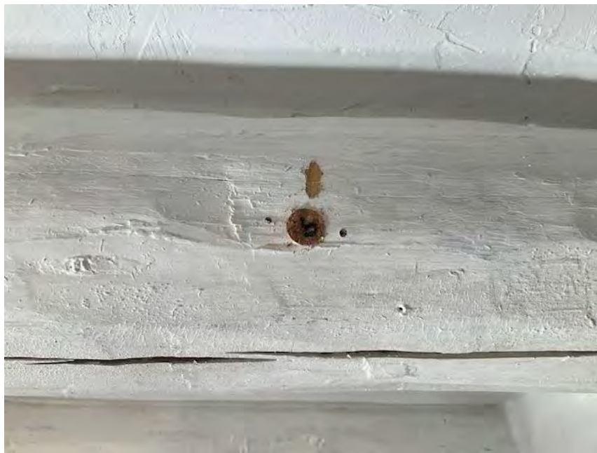
Fig. 4. Increment core hole in one of the ponderosa pine vigas in the northeast addition (Adams 5 or Adams 6). Both vigas yield outer cutting dates of 1922 or 1923, which, like the two interior support posts, suggest the same felling season, implying that the living-room reinforcement and the northeast addition were completed as a single remodeling campaign.
