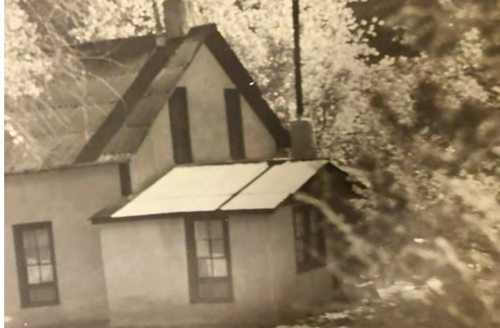
Fig. 10. The Adams House in a ca. 1950s family photograph. The steep gable, the two second-story windows, and the shed-roofed porch are still present today. By the time of this photograph, the 1922–1923 reinforcements and northeast addition had long been in place.
