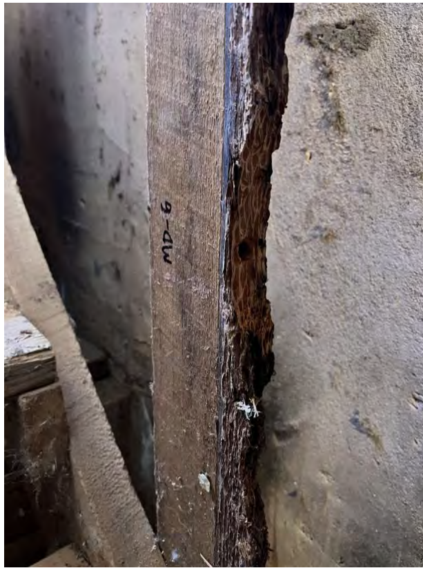
Fig. 2. The vertical stair-support board that yielded core MD-6, with thick bark on the right side.
